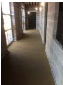
Screed Flooring Ground Floor
