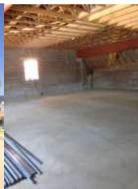
Wessex Hall Screed Flooring Laid
